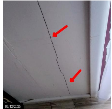
Re-fixing, painting and patching will improve defect noted.
